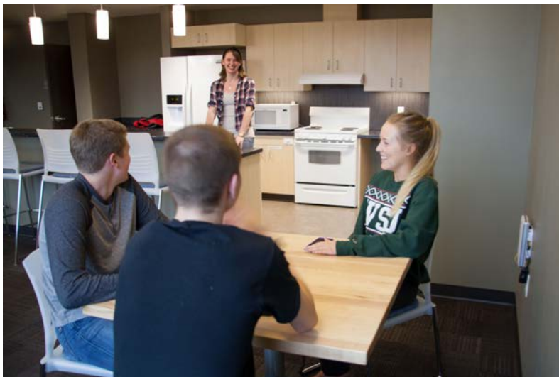
Students can use their connected devices anywhere in the common areas, as well as individual rooms. DASAN Zhone Solutions 2400A, 2600-series, and 2804P GPON ONTs connect each student’s room and public study space to the OLT in the technology closet.
